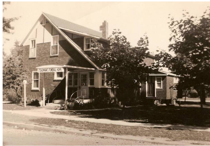
1950s. The small light standard has a cross painted on the glass globe which indicated that ambulance service was available. Photo credit: Andrew Steadman.
